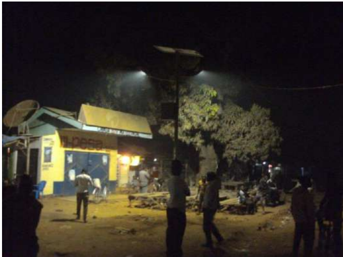
Photo 3: Malinyi market illuminated by solar light ©TAREA
