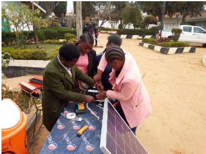
Photo 11: Girls practicing solar home system installation in Njombe © TAREA
