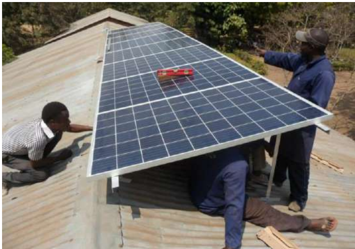
Photo 1: Solar artisans installing a solar system at Igawa Secondary School, Malinyi ©TAREA
